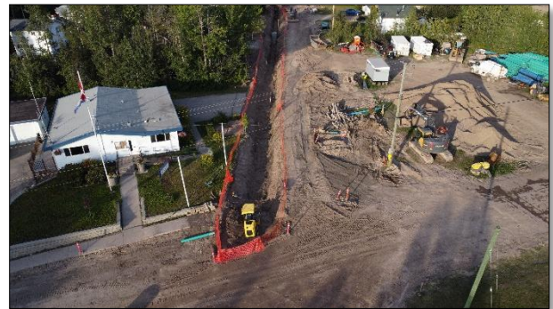
Photo 1 Designated Water Line Construction
