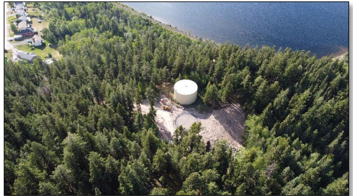
Photo 2 Water Reservoir Construction
